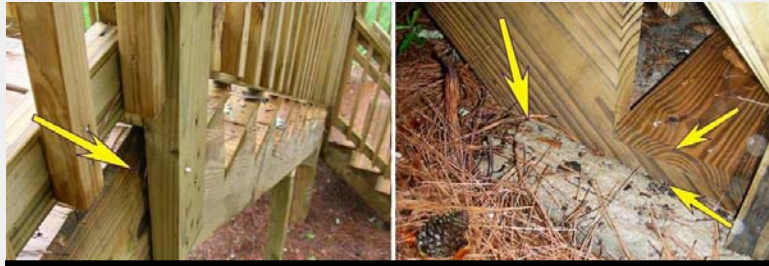
Very Loose Post / Low Step /Ground Contact
