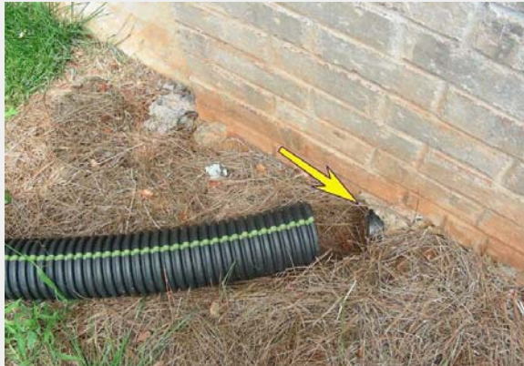
Short Foundation Drain
