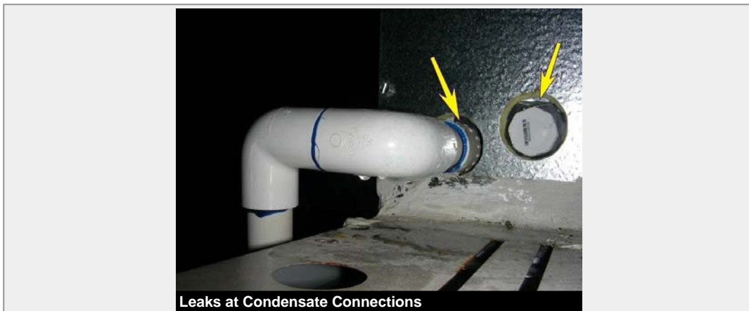
Leaks at Condensate Connections
