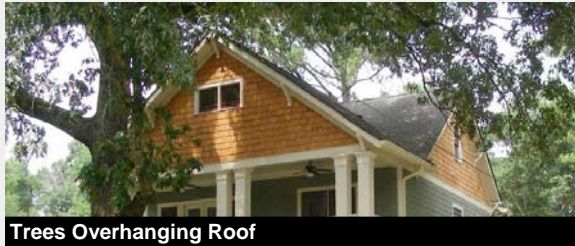
Trees Overhanging Roof
