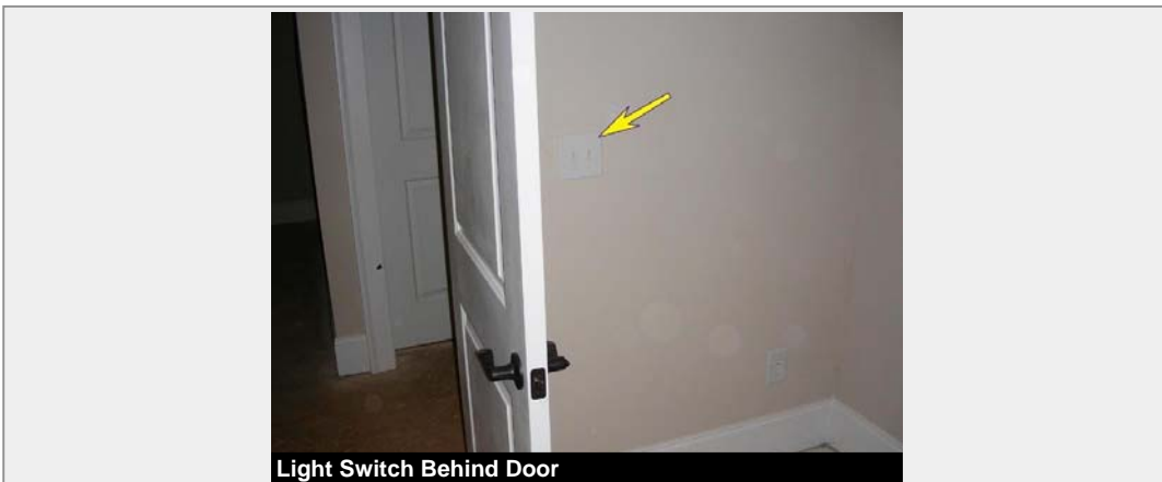
Light Switch Behind Door
