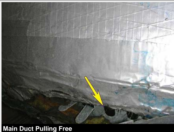
Main Duct Pulling Free
